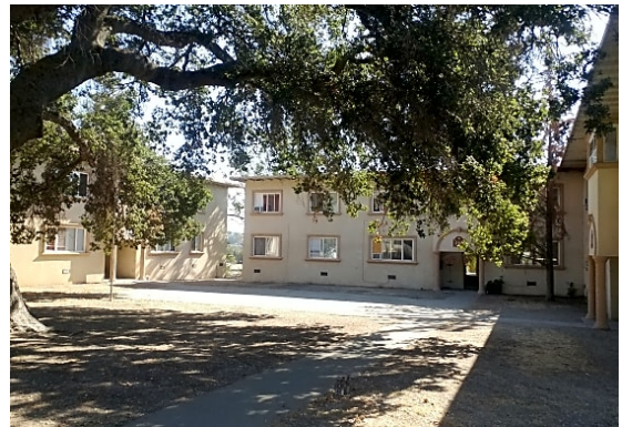
Grand View Apartments. The neglected, mold and vermin infested 54-unit complex at 202 Spring Street, Paso Robles
